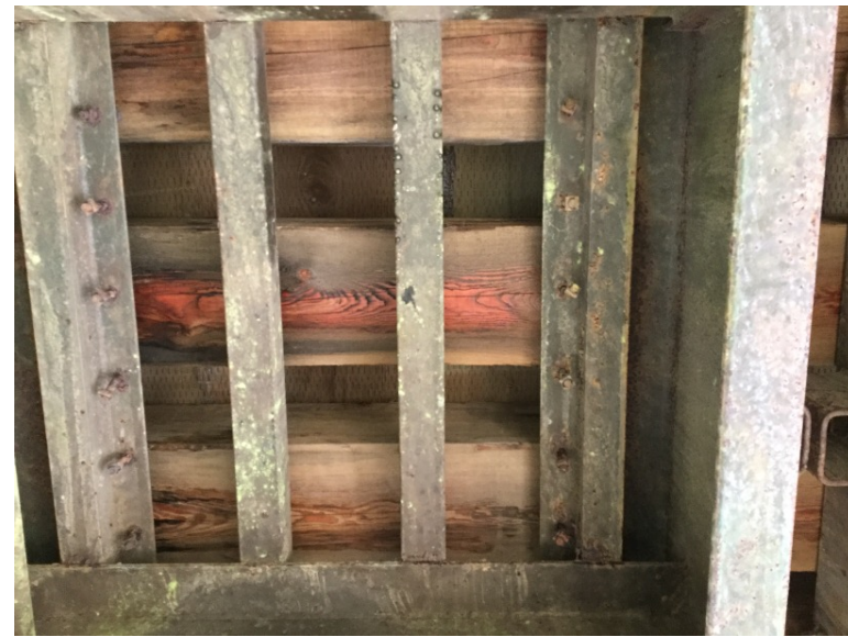
Deck from underneath
