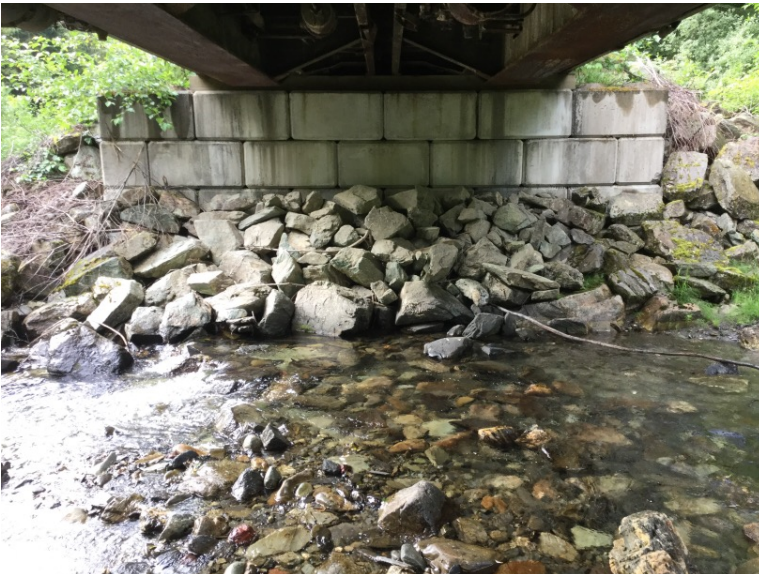
Right Bank Abutment when facing downstream
