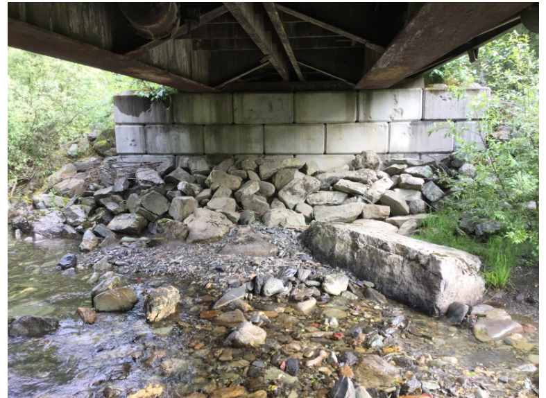
Left Bank Abutment when facing downstream
